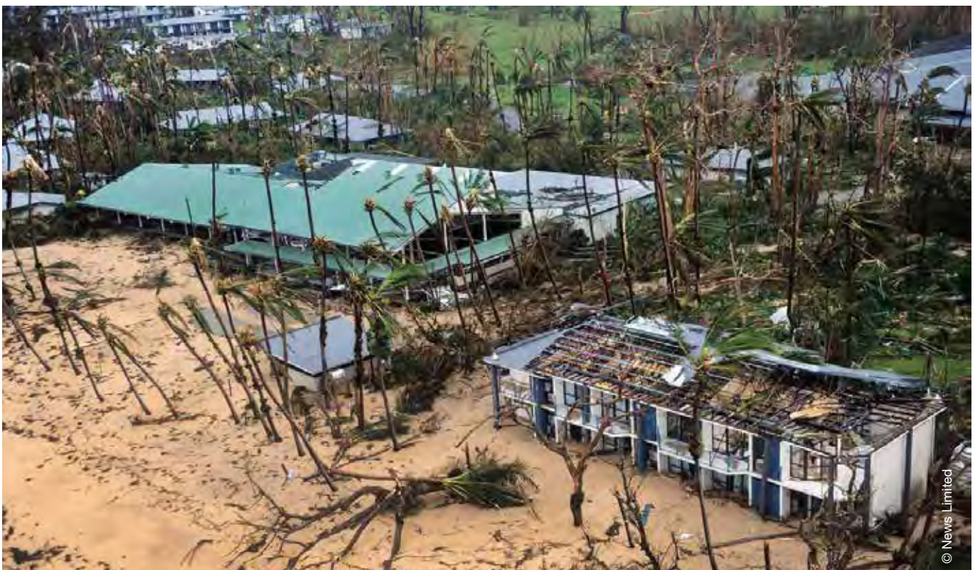
Damage and mass sand deposition at Dunk Island Resort caused by several metre storm surge during TC Yasi.
